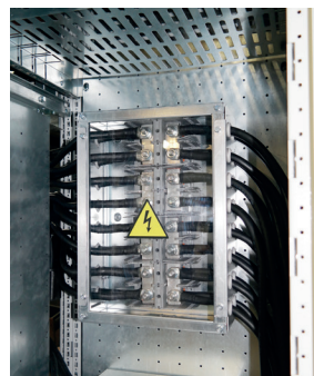
IPXXB finger-proof barriers at cable terminals covering entry.
